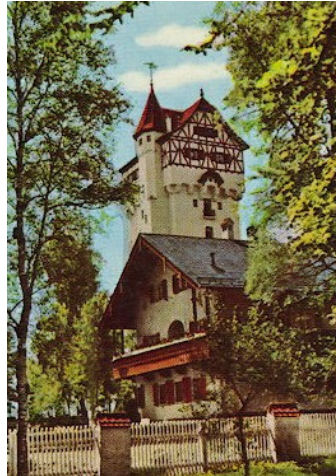
Grafenwohr water tower
