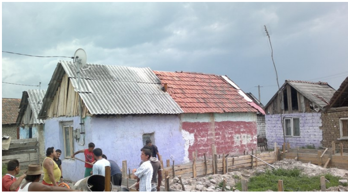
Example of recent improved home construction
