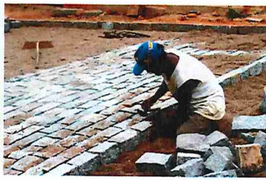
Getting a new street in front of our house.
