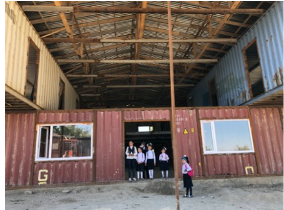
Container school in Tajikistan
